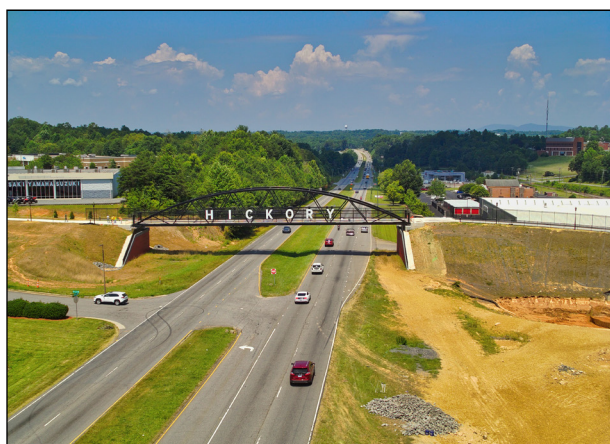
Figure 7: Hickory Trail Overpass on US 321
