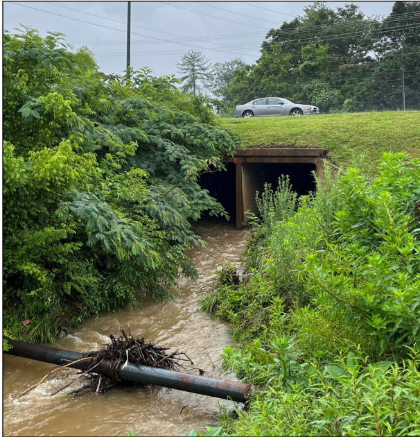
Figure 4: Frye Creek During a Rain Event
