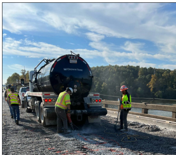
Figure 1: Rehabilitation Work on US 321 Southbound Bridge over the Catawba River
